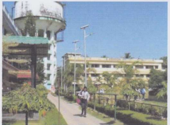
Pic 3 : Installation of Solar Cell on the roof and Solar street lights
